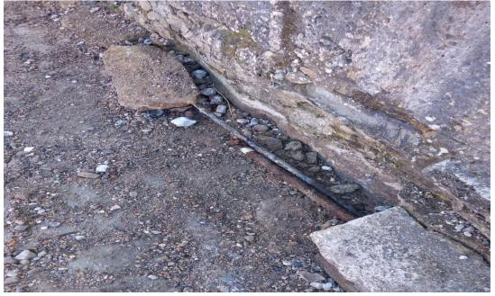
In May the power cable in a different location shorted out and caused sparks to come from the Cobb surface, this left the building without power while National Grid were called to come and repair the damaged cable. This is about the 5<sup>th</sup> time this cable has failed in this way in recent years emphasising the need for the new ducting and upgrade as part of the Phase 5 works.
