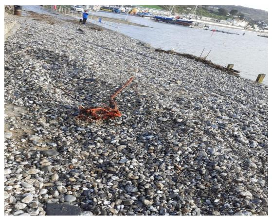
Stone and wave action also exposed the power cable that supply's all the Cobb buildings
